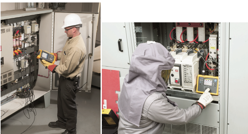
Fig. 5. Measuring in an installation requires several safety measures (Source: Fluke).
